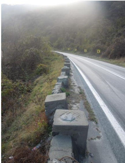
Fig. 9 - 10 Elemente constructive aflate in stare avansata de degradare
